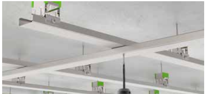
10.- Place transverse profiles in position.
