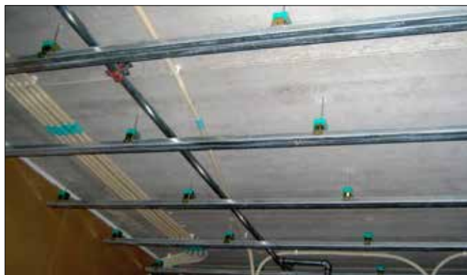
Application of an Akustik Super T60 +Sylomer 30 type B.
