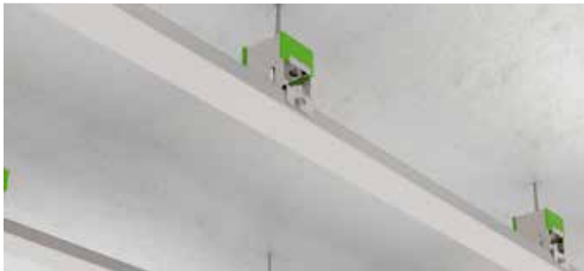
9.- Acoustic hangers and profiles fixed.
