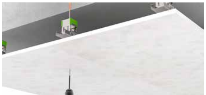
12.- Position plasterboards in place.
